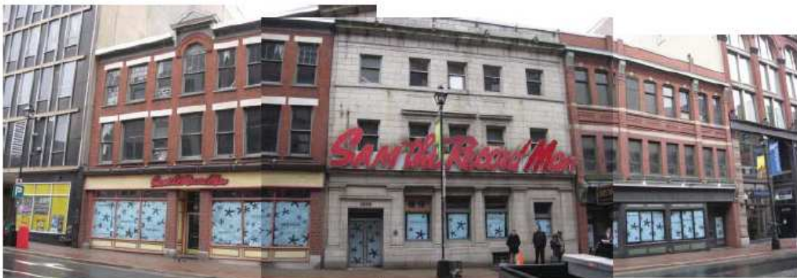
Existing Buildings, 1652, 1656 & 1662 Barrington Street, Halifax, NS
